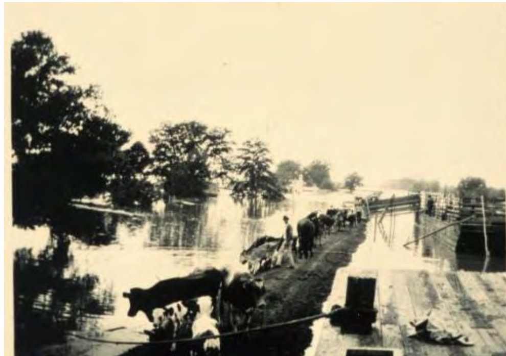
NOAA early flooding along a levee
